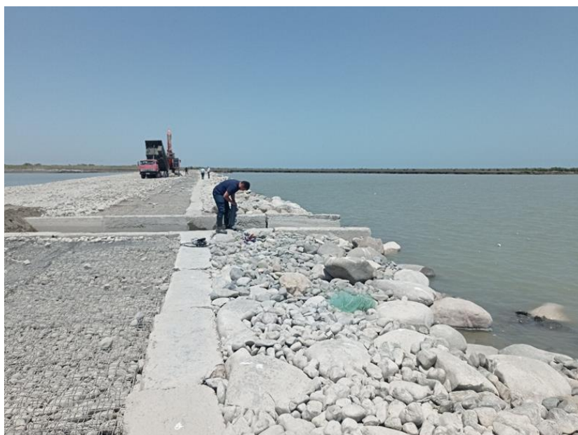
Figure 4: Construction works in 2023 in the Ana Kura branch to prevent seawater intrusion
